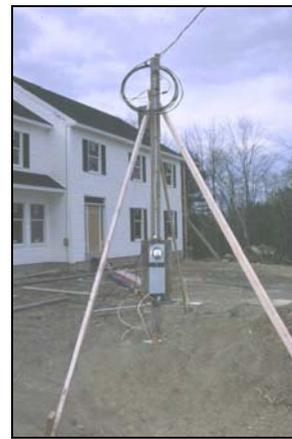
**Figure 5: Temporary Power Distribution Setups**
